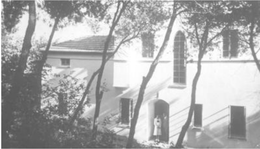
Figure 4.1: My parents, standing in front of their house in Beirut. It had been an old and somewhat decayed Arab house. My father had it rebuilt and enlarged with the help of an architect named Russell Larken.
